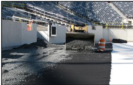
The Meadowlands Stadium is the newest NFL stadium to install a synthetic turf playing surface. Construction at the site was complicated by poor surface conditions and required a solution that provided excellent drainage, high compressive stiffness to support traffic, and high tensile
